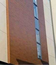
Decoral is a heat transfer sublimation process that has been in our Cork facility since 2005. It is a process where we apply a wood like or other surface finishes such as rusted or stainless steel effect to our aluminium profiles and sheet metal. We also apply bespoke finishes if the quantities are large enough
