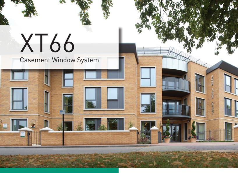
The XT66 'Energy' Casement Window System has been developed to further enhance the performance and energy efficiency of our window suites. It is eco-friendly, sustainable, fully certified, patented aluminium window system. Measuring 66 mm in depth. It can be glazed both internally or externally with 28 mm through to 48mm units with a range of sash styles. The XT66 is fully compatible and interchangeable with the TS66 & XTC66 window systems.
